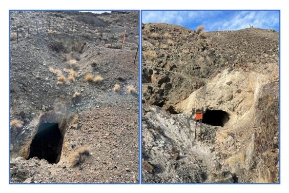
Photo 2 (left): Open stopes along the NW Montreal veins, southern end. Photo 3 (right): Highly altered, mineralized zone at the NW Montreal mine site. One of many such workings.
